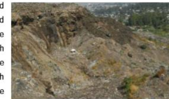
Landfill collapse in Addis Ababa, Ethiopia
