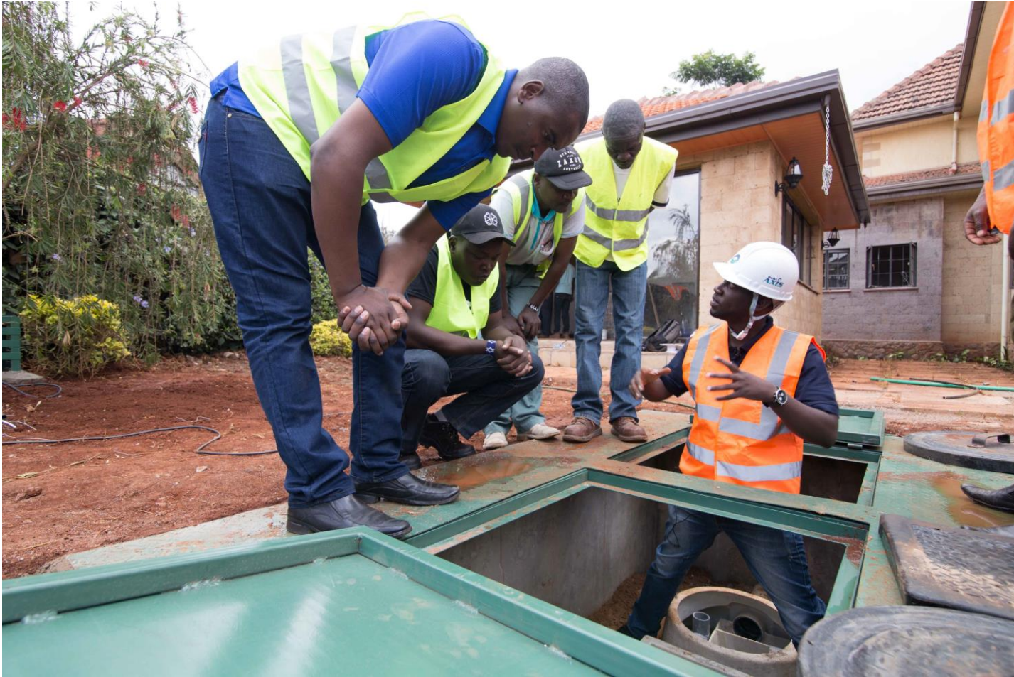
Training for Kenyan plumbers at installation site
